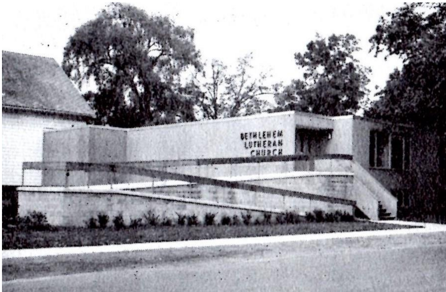
Handicap Ramp to Parish Education Wing 1971
